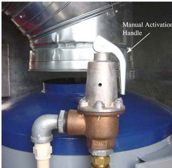
Fig. 4 Temperature and Pressure Relief Valve
