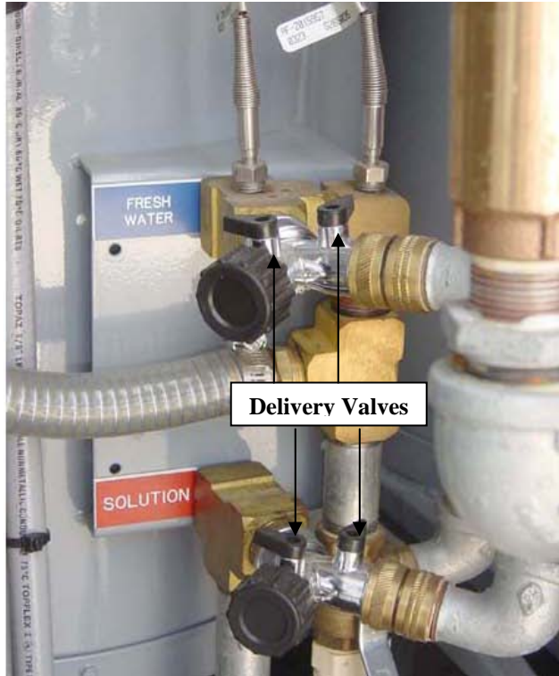
Fig. 5 Water Heater Delivery Valves
