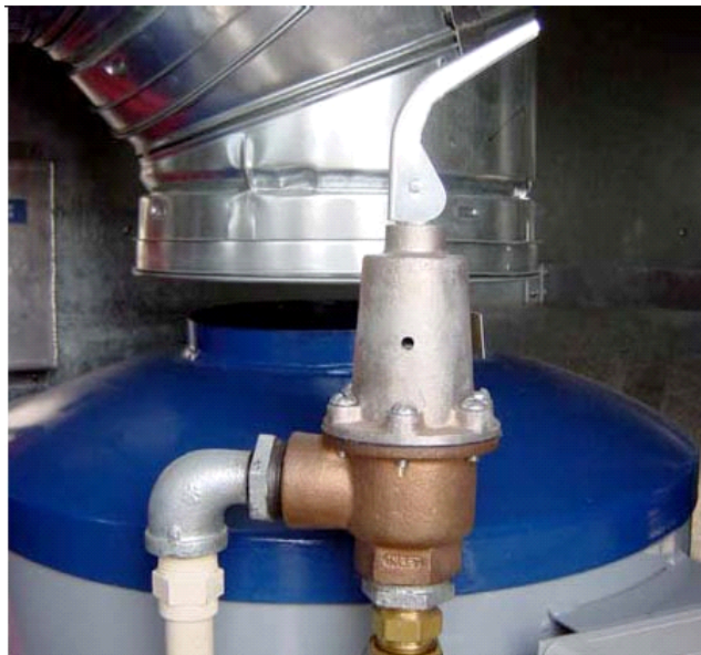
Fig. 6 Temperature & Pressure Relief Valve - Open
